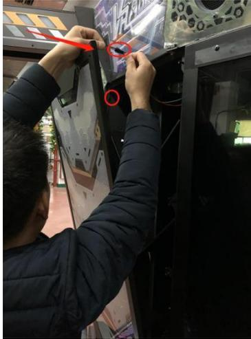
37. Fix the middle frame assembly to monitor cabinet with screws.
