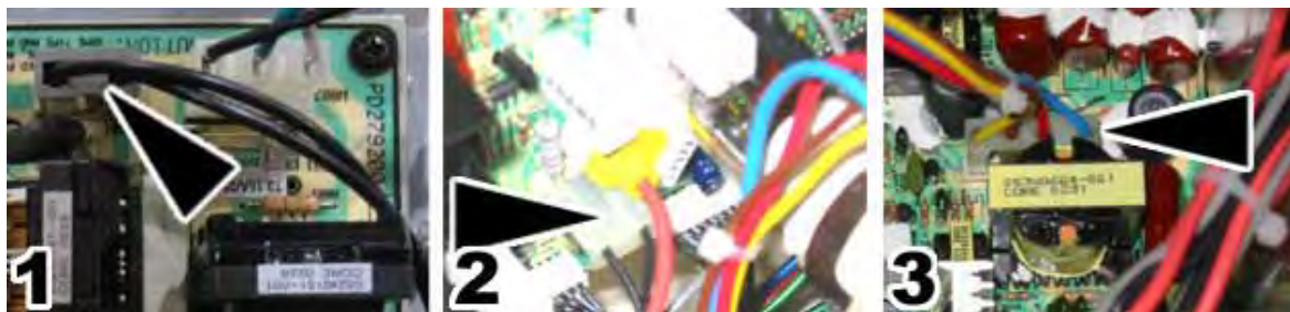
Figure 28. Monitor PCB Cables
