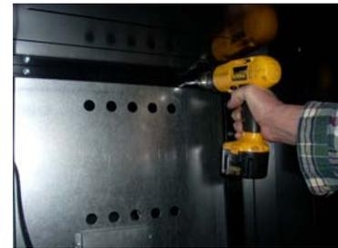
1. On a soft surface, lay the main machine on its front face (front has LED timer). With an assistant, position the base as so the flat front and back sections of the base are in the up and down position. Fasten the base to the machine by aligning the holes in the base with the holes in the bottom of the main machine and attach with (8) 1/4 X 1" self threading screws (fig. C).
