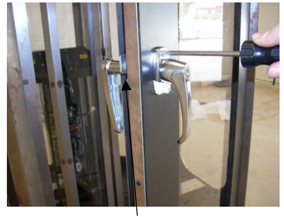
assemble in locked position as shown
