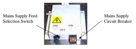
Should this device trip, firstly ascertain the cause of the fault and rectify. To reset the device, simply depress the yellow centre back into the body of the circuit breaker.
