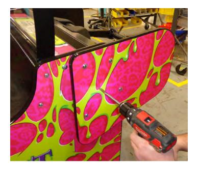
**STEP 9:** remove left side wing and attach middle wing with the same screws that you took out
