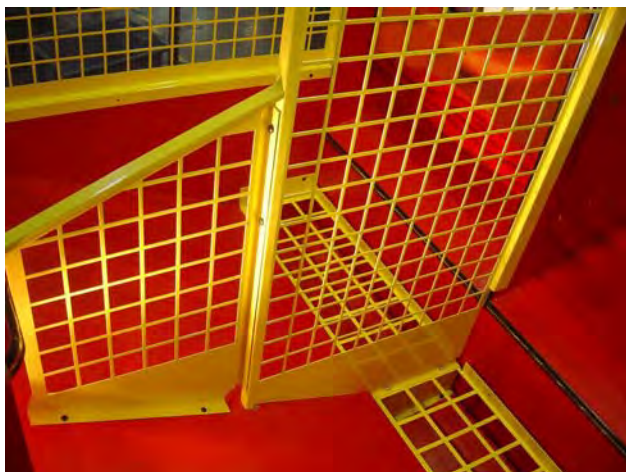
Figure 7 Installing Middle Screen
